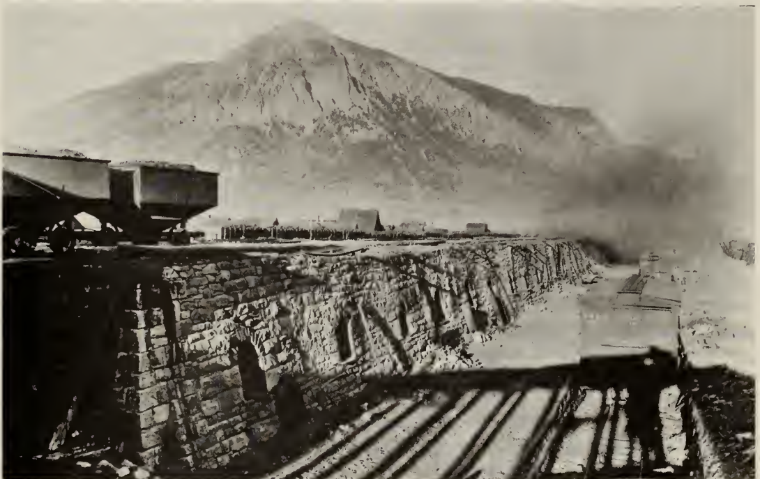
Coke Ovens at Crested Butte Denver Public Library, Western History Division
